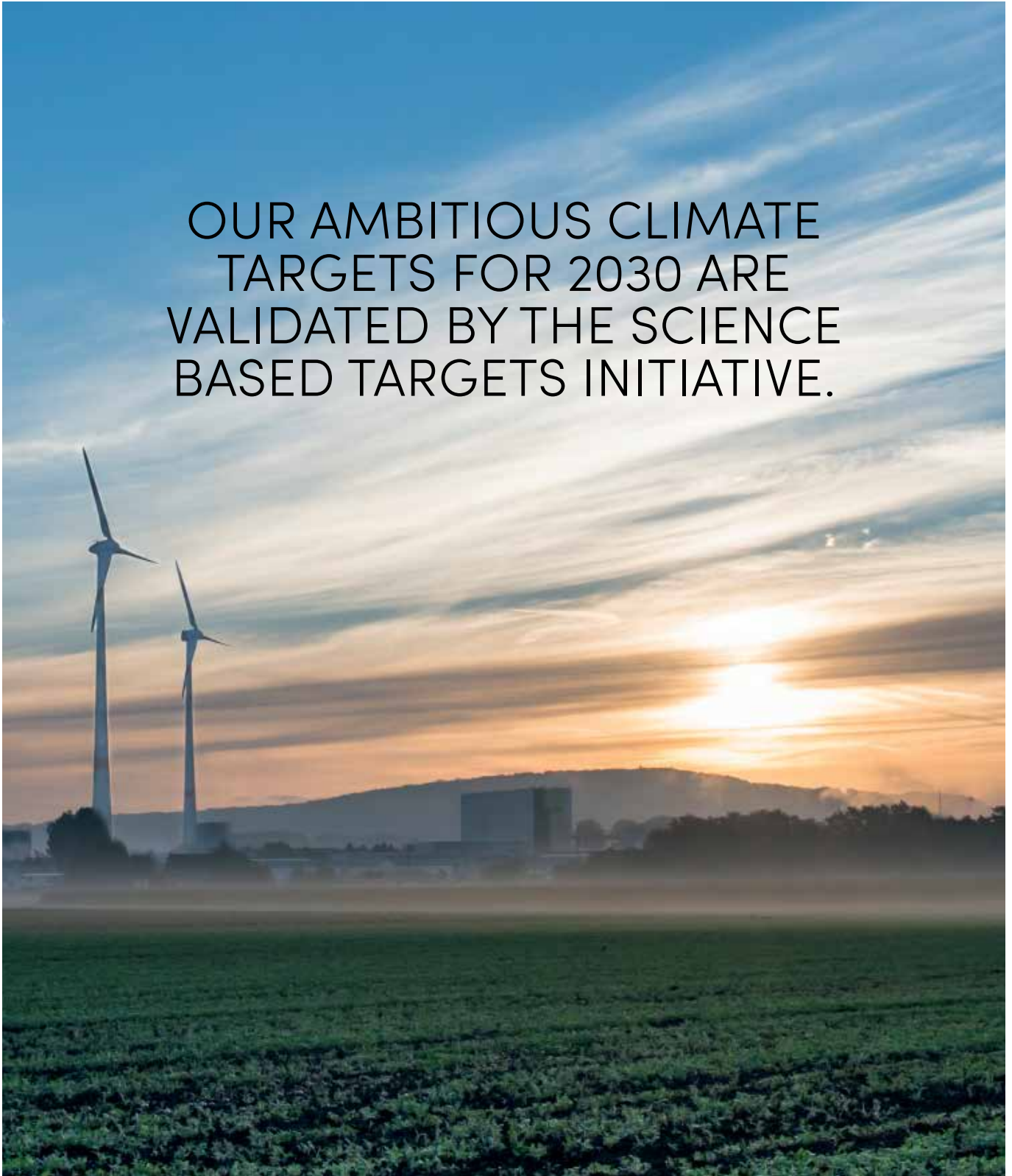
Windmills at Unilin production plant.
